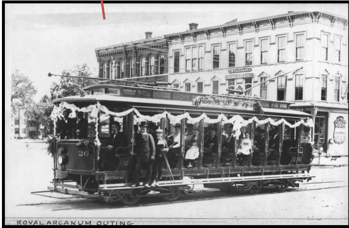
Henry Block (21 South) — Central Block (1-3 South)
