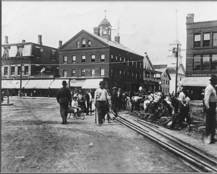
LAYING TROLLEY TRACKS 1903
